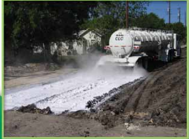
Lime Being Applied
