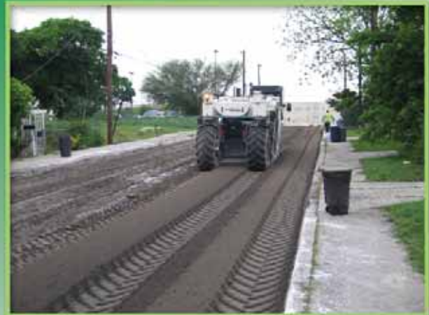
Mixing of Lime Stabilized Soil
