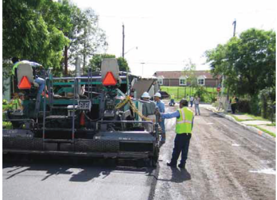
Photo 5: Warm-Mix Asphalt being Placed on Maryland Street
