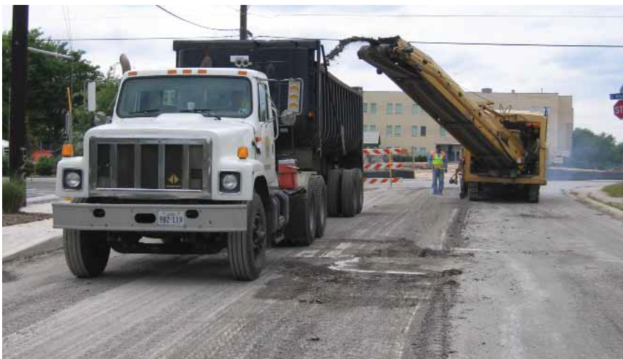
Photo 1: Milling of Existing Roadway on Maryland Street
