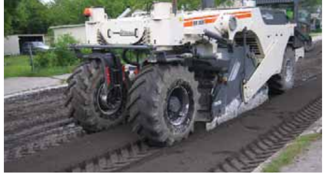
Photo 4: Notice Change in Soil after Lime Breaks Down the Clay and Makes it a Granular Material
