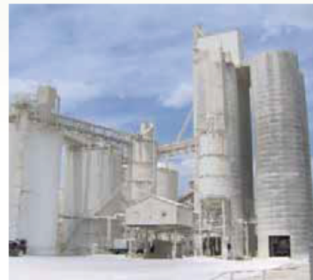
Texas Lime Product Silos
