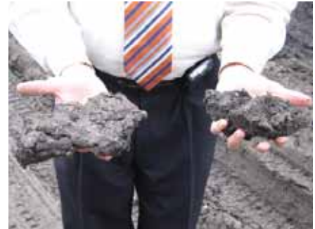
Photo 2: Clods of Highly Expansive Clay Found in Subgrade on Maryland St.
