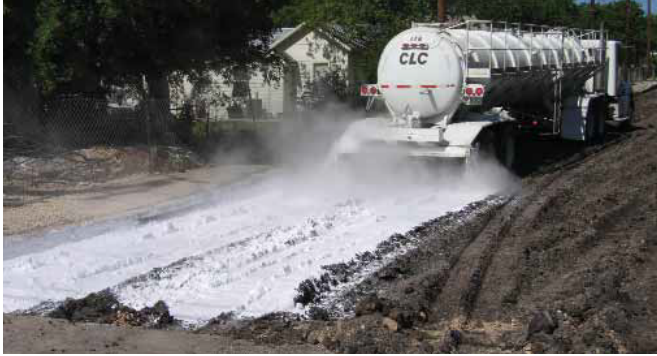
Photo 3: Lime Slurry Placement on Clay Subgrade
