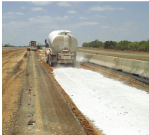
Lime Slurry Being Applied to Subgrade on Interstate 35 Project in LaSalle County, N. of Laredo
