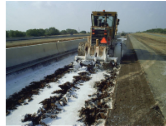
Motor Grader Working Lime Slurry into Subgrade
