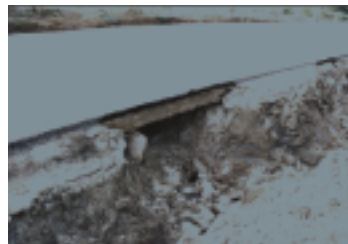
Figure 2. Proper stabilization provides a durable, long-term material as evidenced by this base layer bridging a washed out area.
