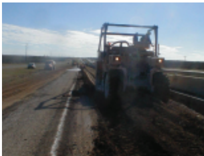
Subgrade Leveling Begins after Lime is Worked In
