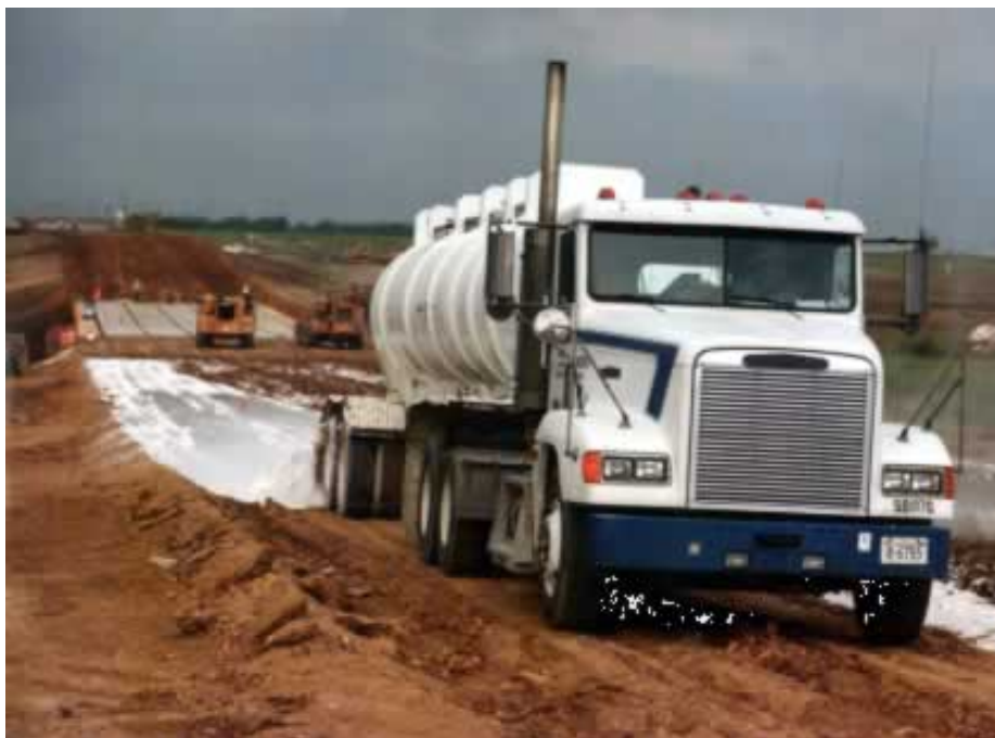
Figure 9: Soil windrow used to contain lime before mixing
